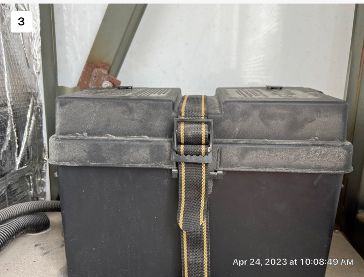
The battery has a battery box with a cover and a strap to secure the battery.
