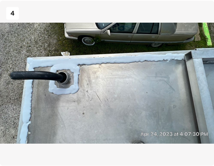
New sealant is applied around the perimeter joints and roof penetrations.
