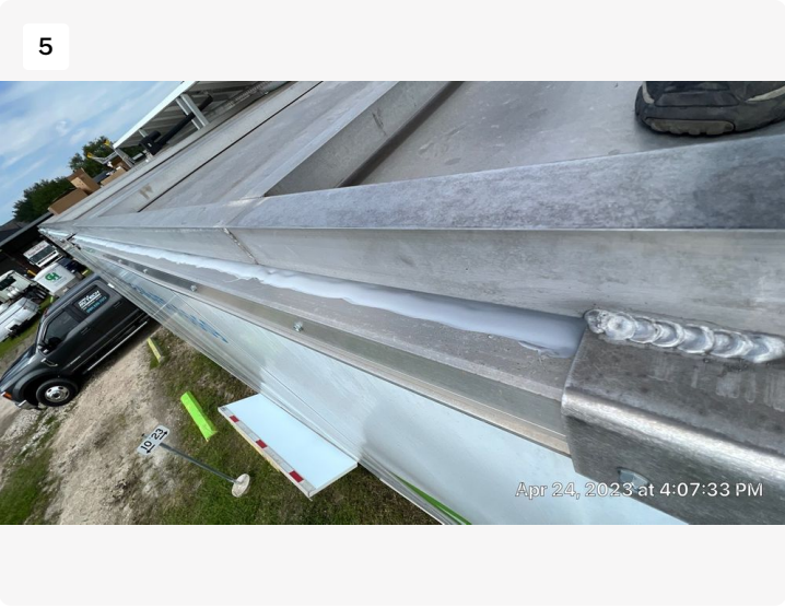
New sealant is applied around the accessible perimeter joints.
