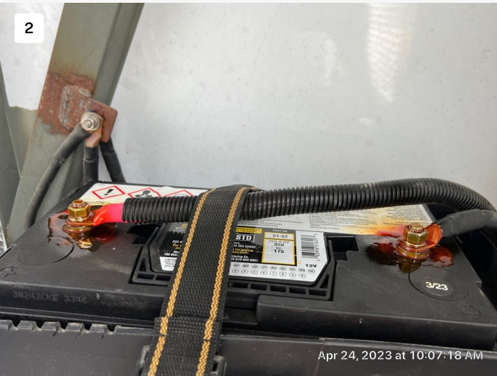
New battery installed with anti corrosion spray applied to the terminals.
